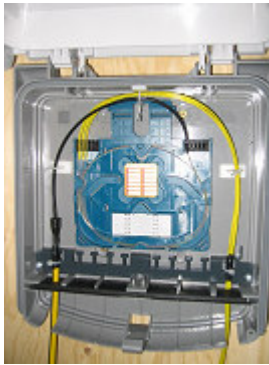
Figure 13. Standard wall mountable 3M box with dimensions (HxWxD): 290x255x86 mm
